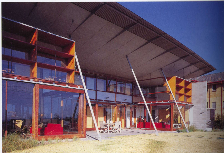
View from northeast: garden 北東より見る：庭
