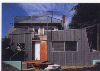
Frank O. Gehry: Gehry Residence
