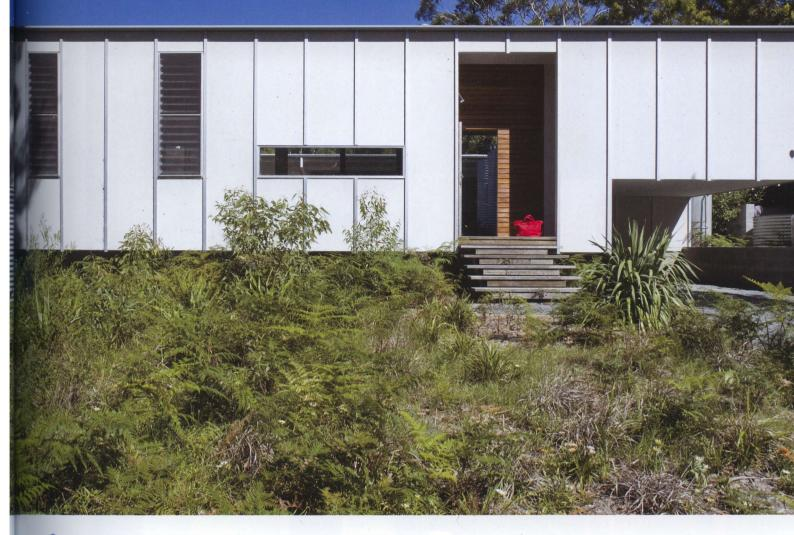
The wall material is compressed fibre cement sheet which is durable, needs no top coat and requires little maintenance. The sheets are fixed with stainless steel screws. The dimensions of the cement sheets were instrumental to the design of the house, which was worked out dimensionally from the width of a sheet — 900mm plus a 10mm gap — reducing
