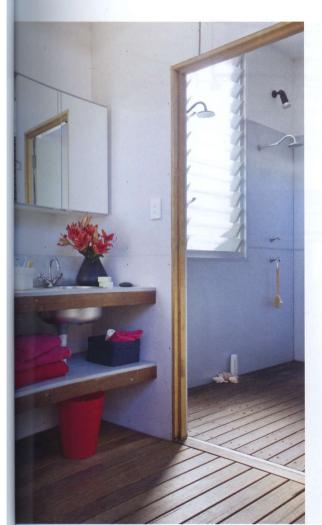
Shelves are made from cement sheet with blackbutt supports. The owners opted for zincalume sheeting behind the showers instead of tiling. The sheets just need a wipe down from time to time, and could last ten to 15 years before needing replacement. The replacement process would also be significantly easier and quicker than that for tiles.
